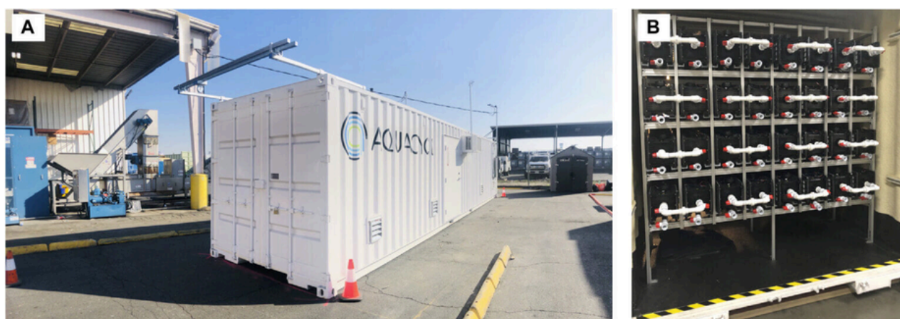
FIGURE 9 | 12-m C-BETT system installed at a soda manufacturer customer site. (A) Outside view of C-BETT and (B) BETT reactors arrangement inside C-BETT.
